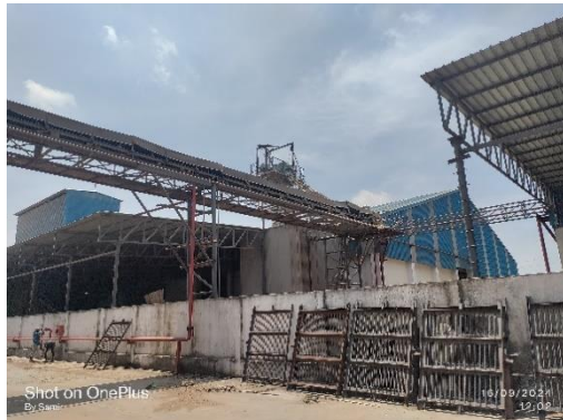
Feed Conveyor to Maize Cleaning
